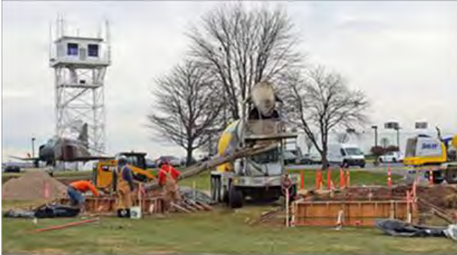
Force Construction Company built the display site.
