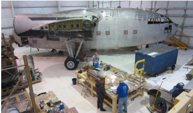
The Restoration Team worked inside a hangar during the winter to clean and repair Charlie 119 components.
